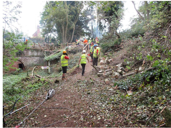
Berwick tunnel . Photo credit James Weir
