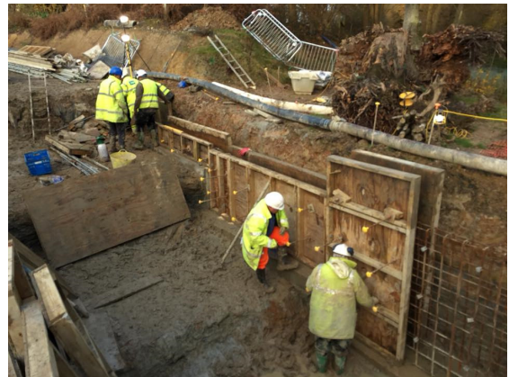
Creating shuttering for the slipway. Photo credit Tim Lewis
