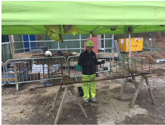
Creating reinforcement for the walls of the slipway. Photo credit Tim Lewis
