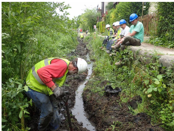
Five to one mix with Martin digging the channel. Photo credit Tim Lewis
